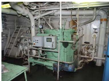
Figure 1 - Typical OWS – does it work? Is the discharge less than 15ppm?
